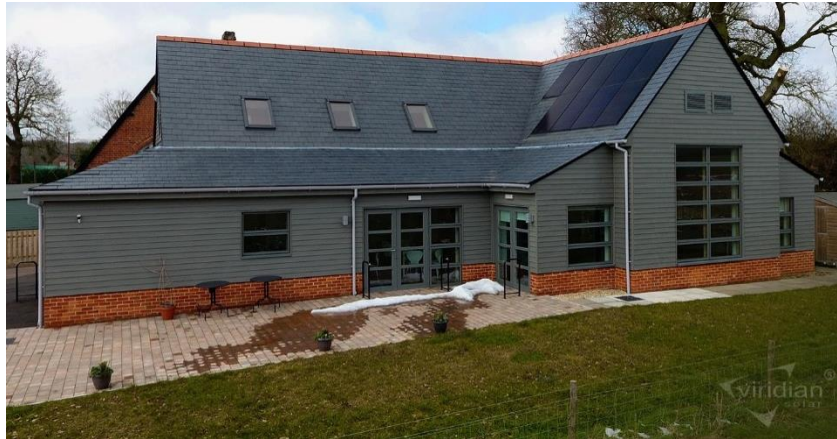
Figure 3: In-roof PV example from Viridian Solar
