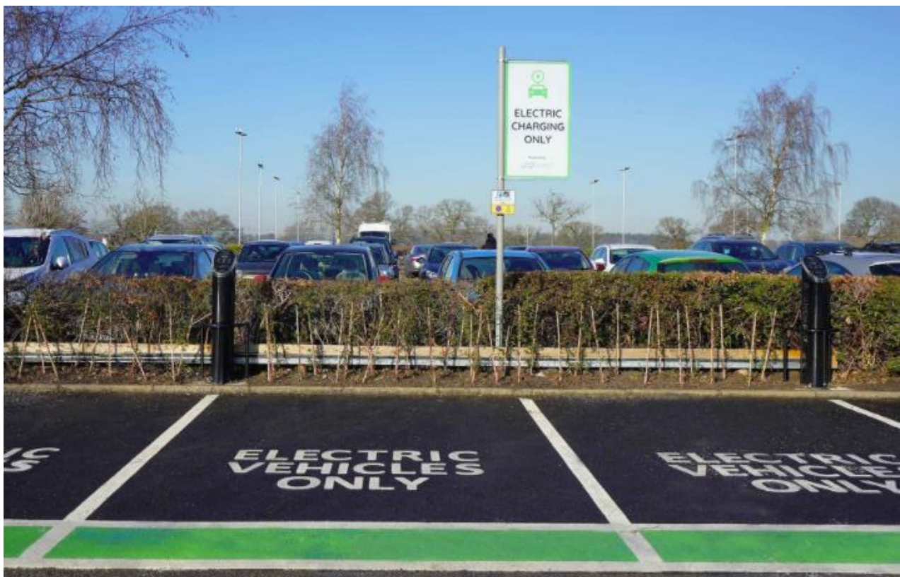
Figure 11: Example stand-alone EV charger 6
