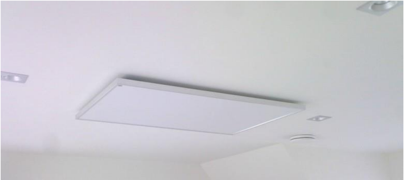
Figure 4: Ceiling mounted infrared heating panel
